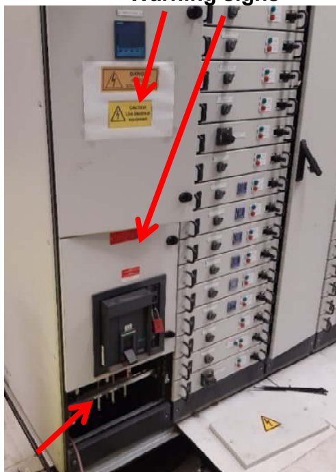
Exposed energized conductors
